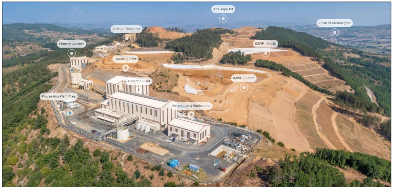
Figure 18-3: Site aerial view
