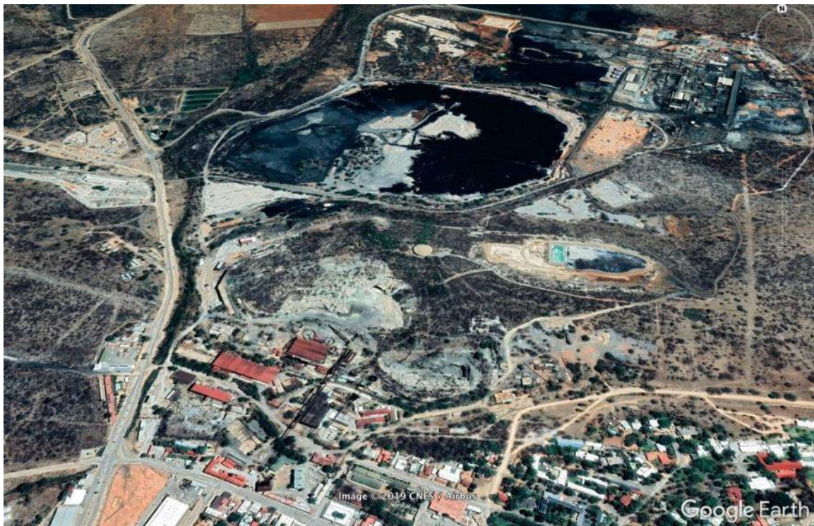
Figure 6: DPMT Smelter and old mine infrastructure seen from the South (Source: Google Earth)
